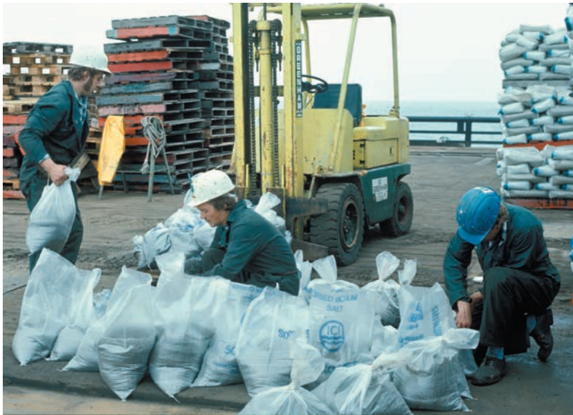
Readying sandbags to cover the gas pipeline from Ekofisk to Emden.
