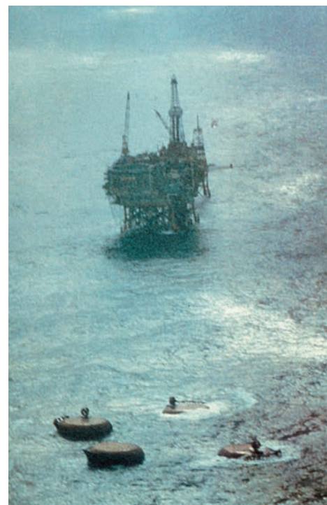
After it had capsized, all that was visible of Alexander L Kielland on the surface was the four remaining pontoons. DSVs Seaway Falcon , Seaway Eagle and Tender Power searched the area. The Edda platform is in the background. Photo: Børre Børretzen
