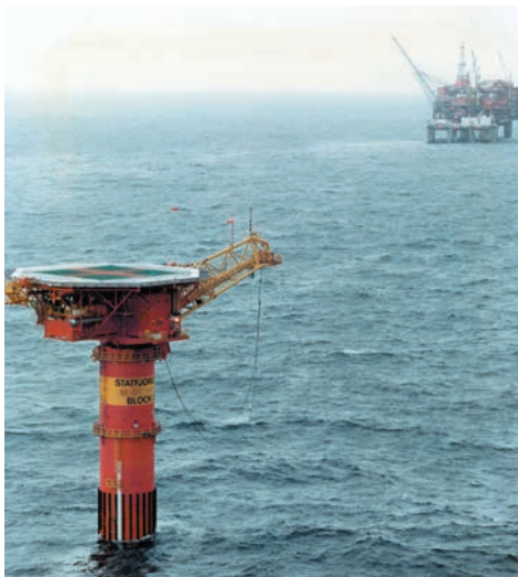
When the Storting dropped the proposal to pipe Statfjord oil across the Norwegian Trench, it was decided to load this output into tankers via buoys on the field. Divers had to make extensive subsea modifications before the system functioned.
