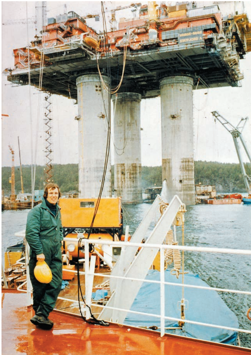
A diver on the diving vessel for Statfjord A at Stord.
