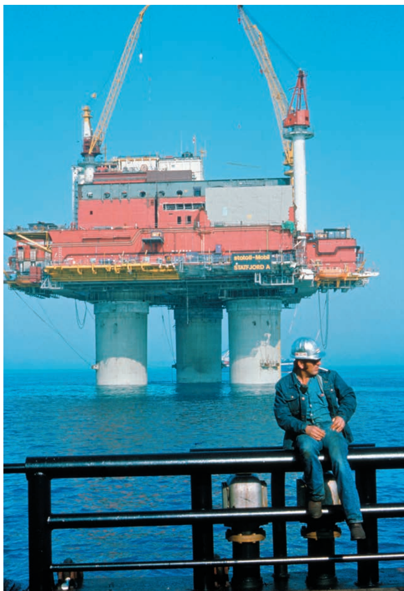
Construction of Statfjord A was a difficult period. Much of the work had to be done after the platform arrived on the field. Life for those involved could shift between waiting and hectic work. The same applied under water. Photo: Leif Berge/Statoil
