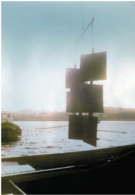
Hoisting steel plates. Photo: Leif-Tore Skjerven
