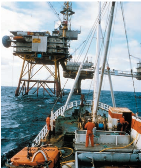
The Snurre ROV carried out cleaning and inspection of three concrete platforms on Frigg during March 1980.
