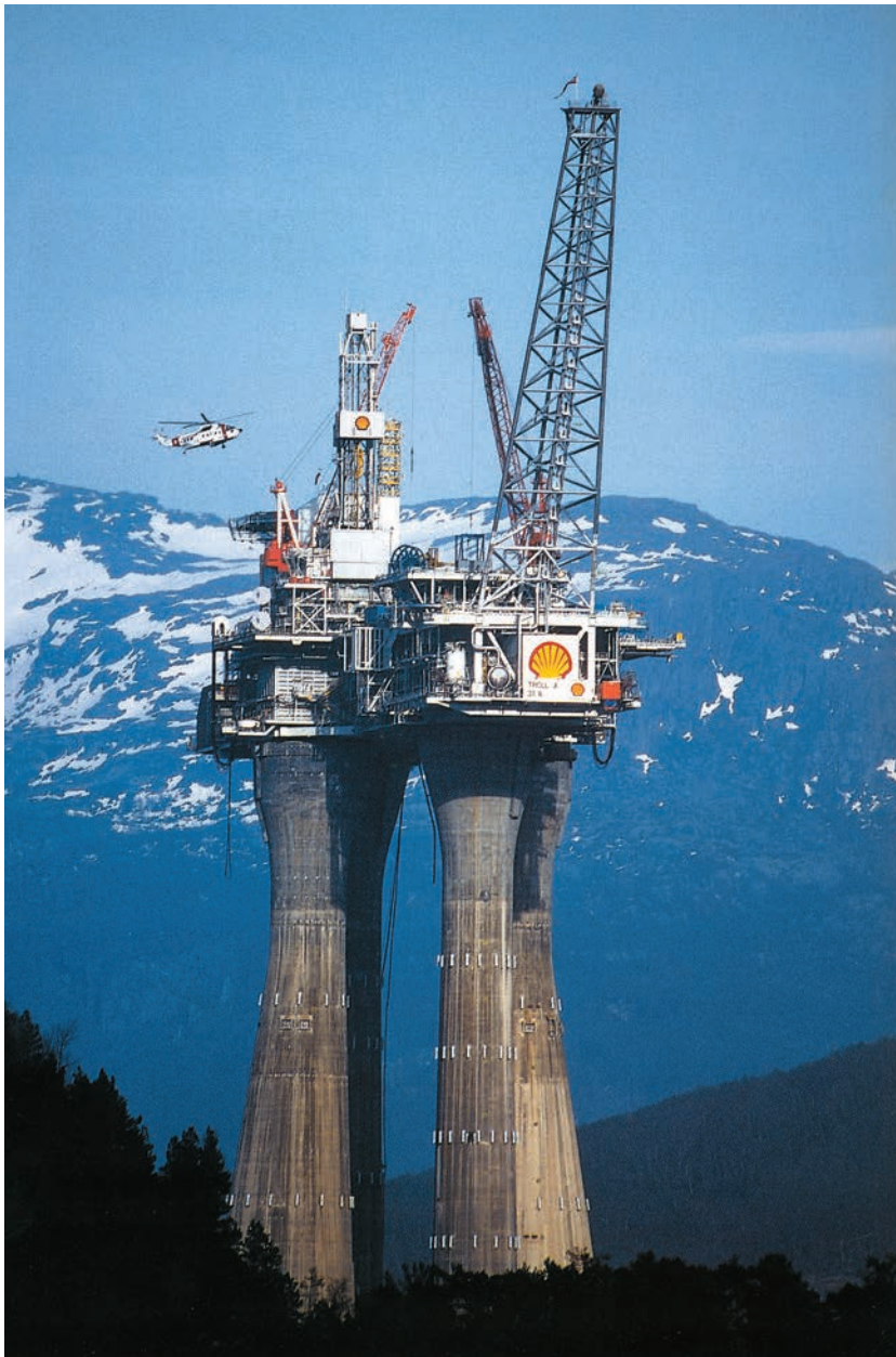
Troll A being towed out to the field. This was in many ways a prestige project. The platform was the tallest structure ever moved over the Earth's surface, measuring 472 metres from its concrete "skirt" to the top of the flare boom.
