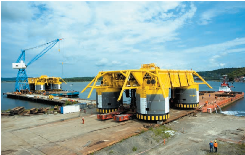
Two giant subsea installations ready for dispatch to Ormen Lange. Each measures 44 x 33 metres.
