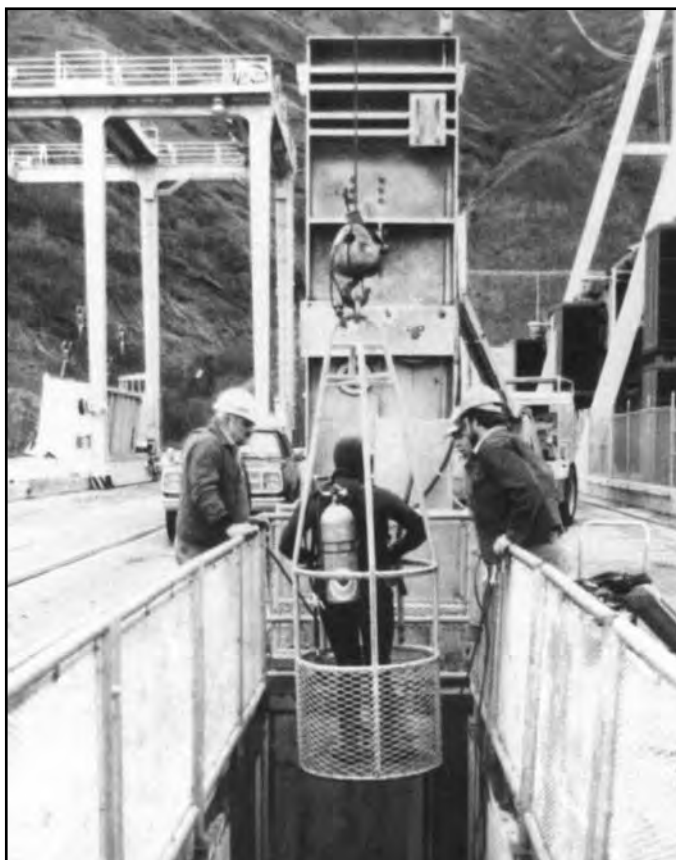
FIGURE 12.15 Line-Tended Diver Lowered into Dam Gatewell
