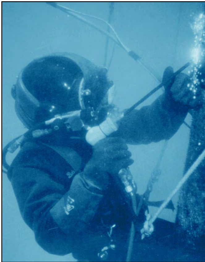
FIGURE 10.16 Ultrathermic Oxy-Arc Process
