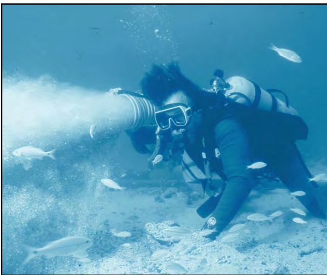
FIGURE 9.45 Backfilling with an Injection Dredge
