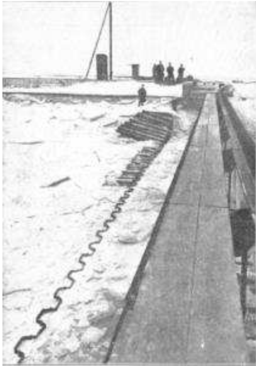
Photo n° 6: Sheet piles cutting 1914 (12)
