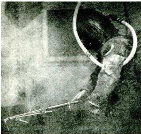
Photo n°44: Cutting test with the 2nd generation Picard AD-8 torch in the Siebe Gorman tank in 1924 (84)
