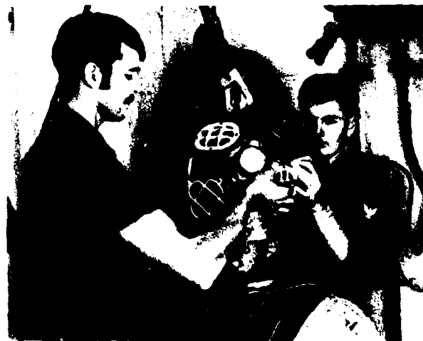
A The helmet, suspended by a small block and tackle, is carefully lowered over the diver's head.
