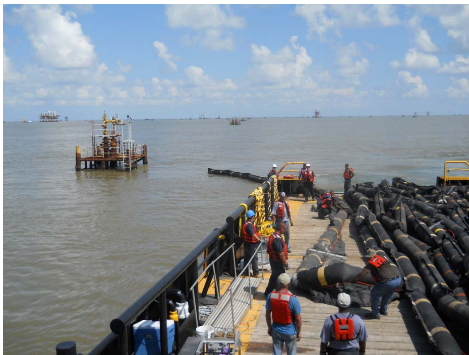
Figure 5-17. Booming Operations off of East Bay, LA on June 22, 2010 demonstrating use of well heads as anchoring point for boom.
