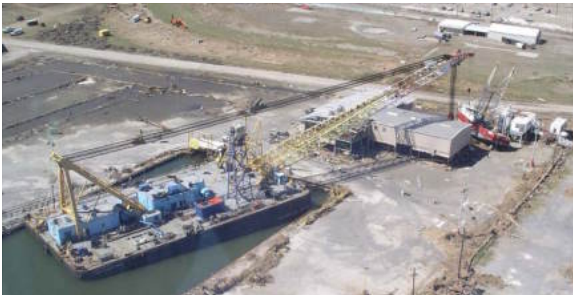
Figure 5-10. Donjon's Chesapeake 1000 working a long-distance lift in Venice, LA.
