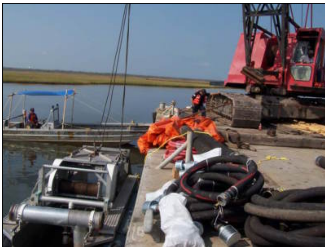
Figure H-8. Crane on Barge Launching the Skimmer
