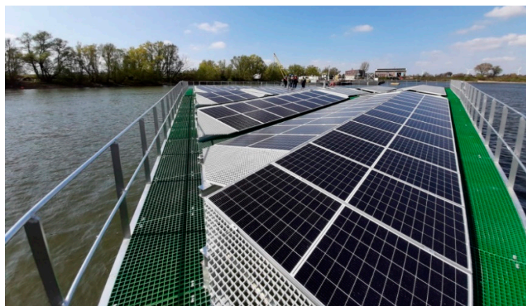
Figure 8. Walkways and fences on the SolarDuck floating offshore platform. Reproduced with permission from authors [45].
