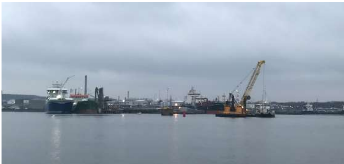
Figure 1. One of the measurements stations in the port of Gothenburg with a dredger (yellow ship) in action. Photo © FOI.
