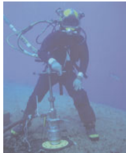
FIGURE 8. LIGHTWEIGHT HOT-TAP.
