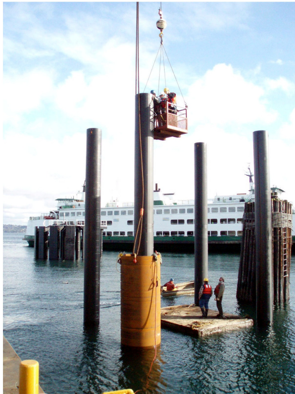
Figure 13. Installation of the TNAP around a 30-in.-diameter pile.
