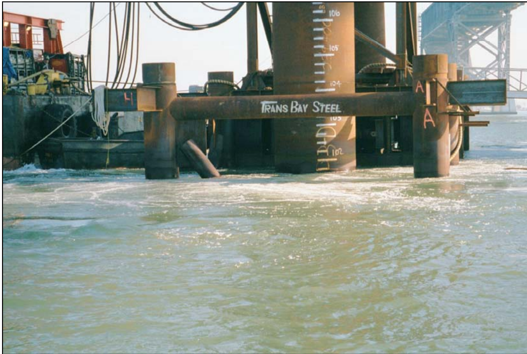
Figure 1-7. Air Bubble Curtain in Operation.
