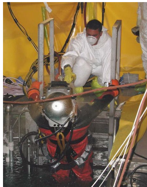
Figure no. 7: Diver supervised by the protection team (Sheaffer, 2015)
