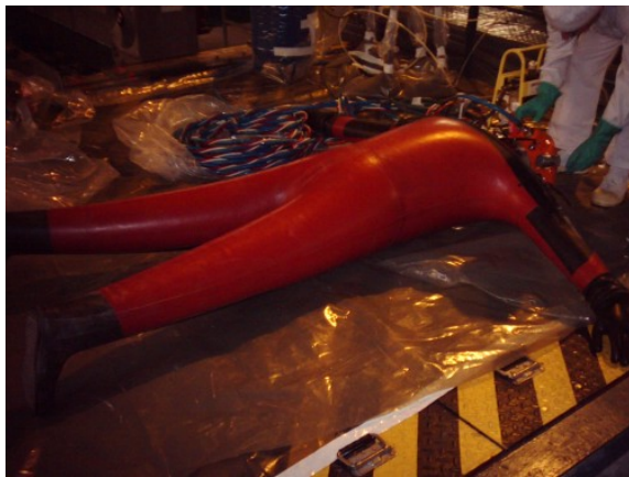
Figure no. 8: Decontamination of the diver after immersion in radioactive environment
