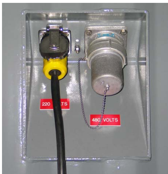
Figure 2-2. Power Receptacle Box
