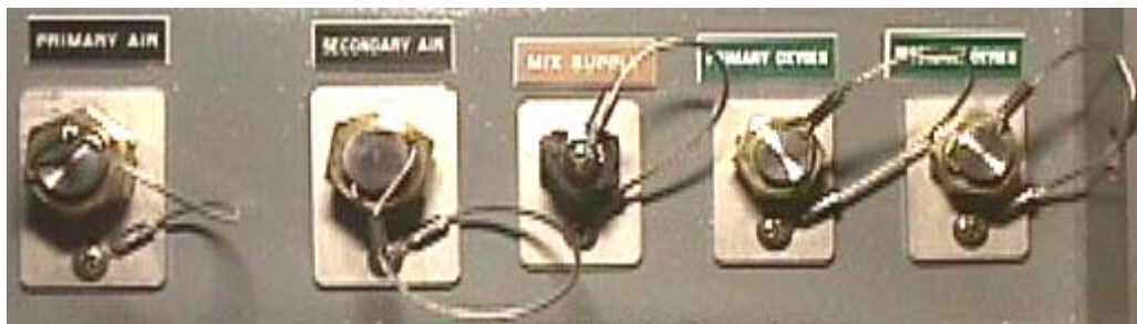
Figure 3-15. External Compressed Gas Supply Connections
