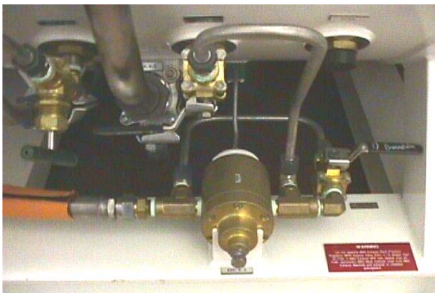
Figure 3-20. BIBS Exhaust Back Pressure Regulator
