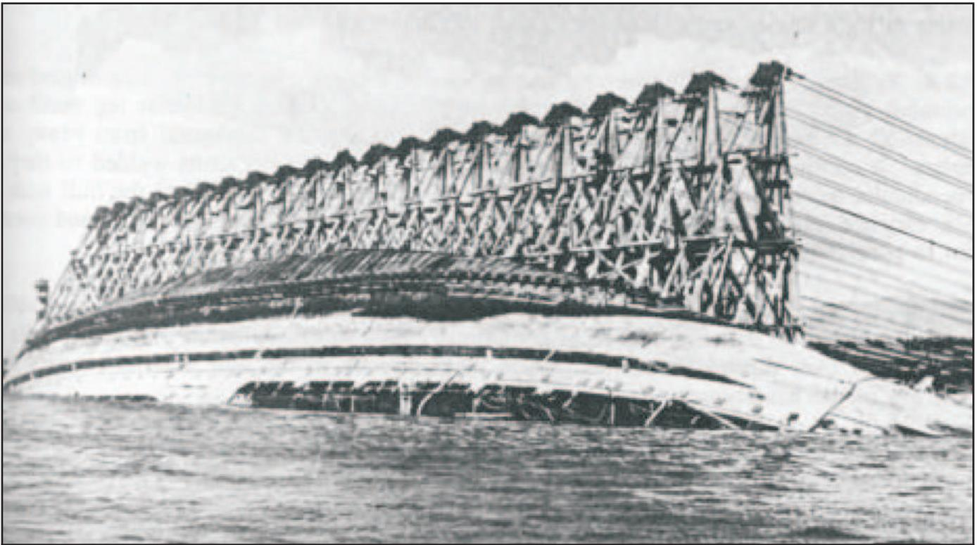
Figure 7-15. Braced-Girder Headframes on USS OKLAHOMA.
