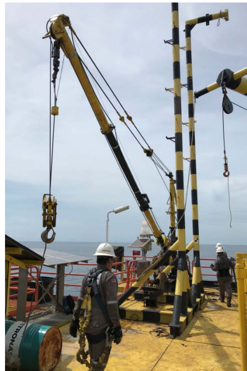
FIGURE 5: PORTABLE CRANE INSTALLATION.
