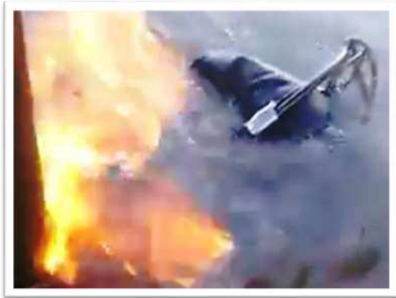
Fig.n° 54: Result of an anode welding against a (rotten) pile containing methane under slight pressure (73).
