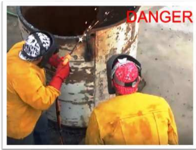
Fig. n° 52: Avoid being in contact with the structure (72)
