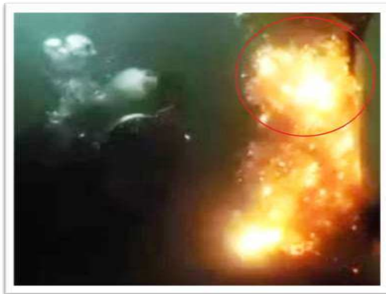
Fig.n°6: Spontaneous ignition of the produced gases (H 2 /CO/other) (5).
