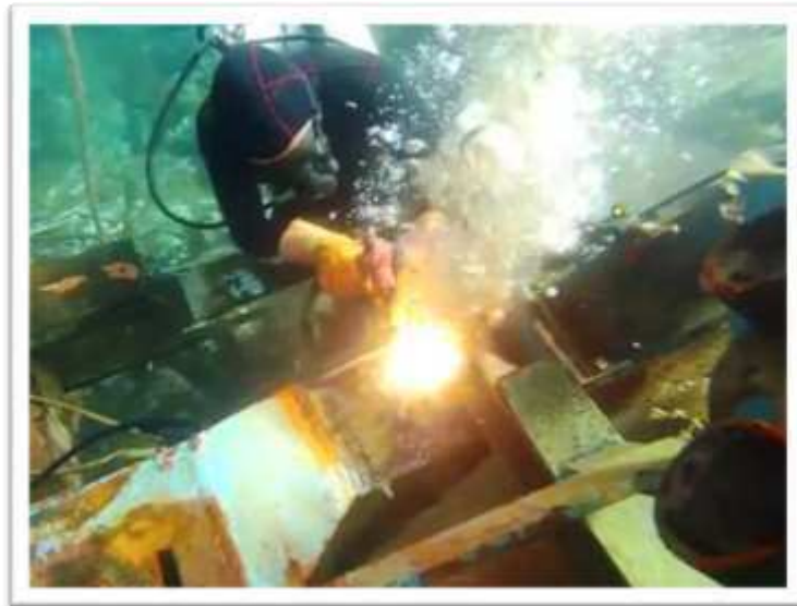
Fig.n° 61: Ultra-thermic cutting with a significant rise of unburned oxygen into the residual gases (82).
