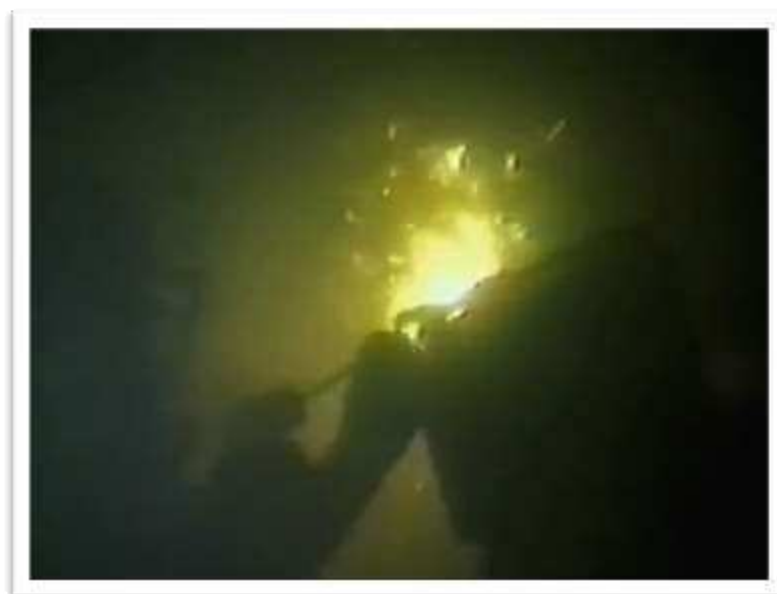
Fig.n° 62: Oxy-arc cutting with a limited rise of unburned oxygen into the residual gases (83).
