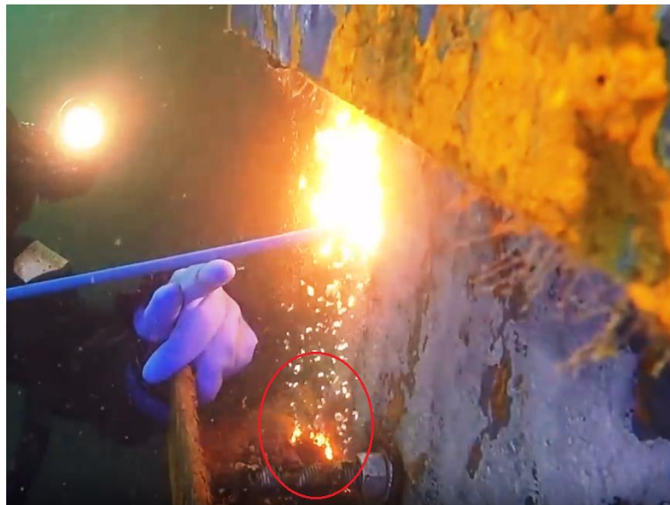
Fig 2: Formation of gas bubbles 8
