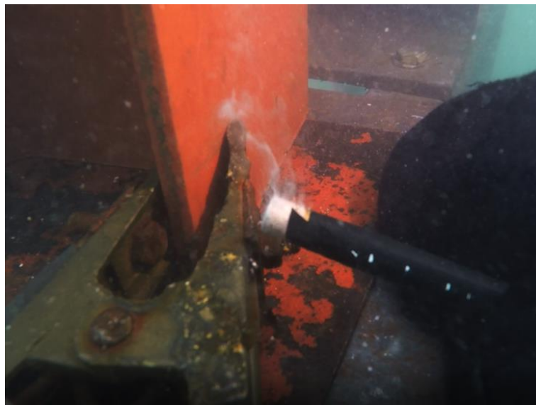
Fig 8: Electrolysis at the back of the rod
