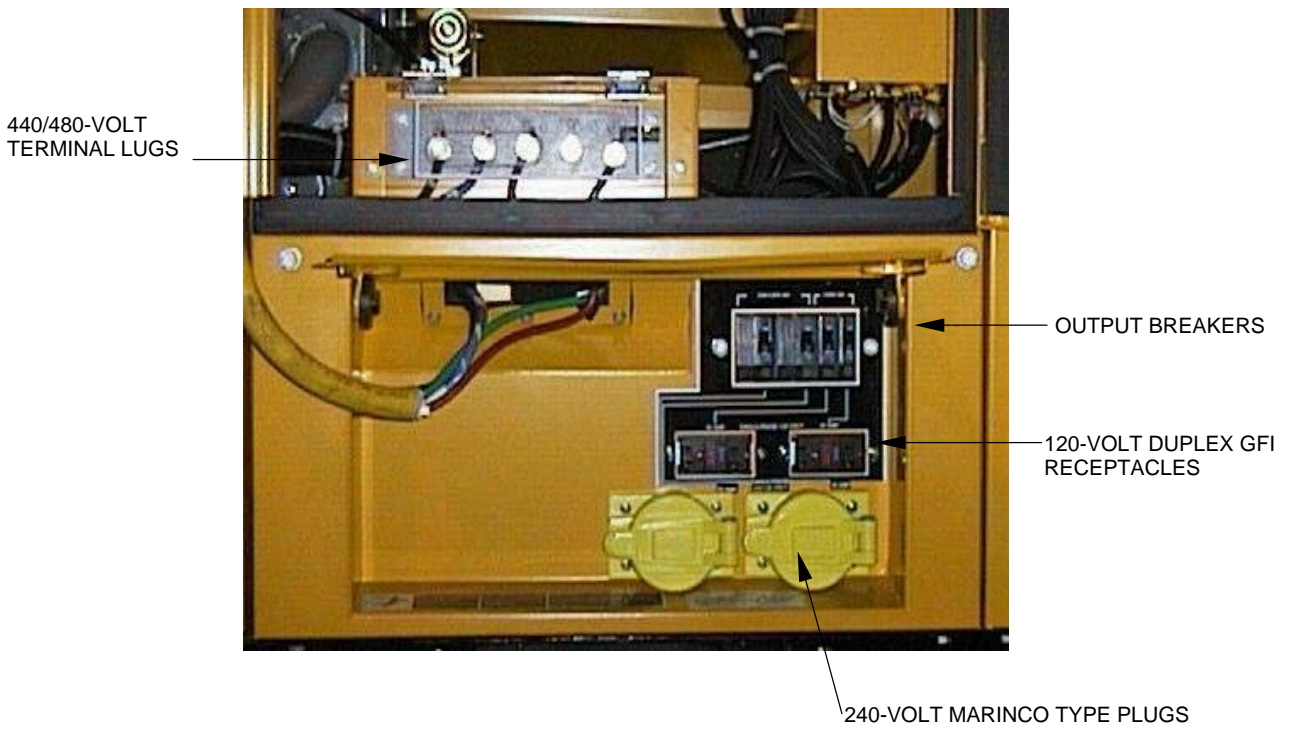
GE0500A Electrical Connections
