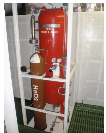
Volume tank & its pressurization sys.
