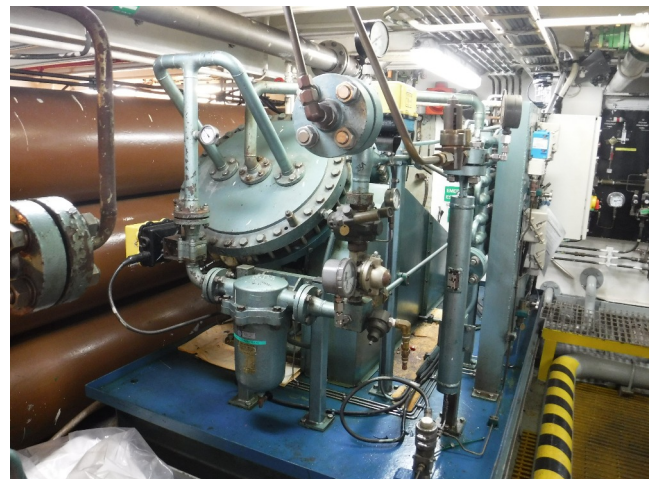
Compressor two stages arranged in "V"
