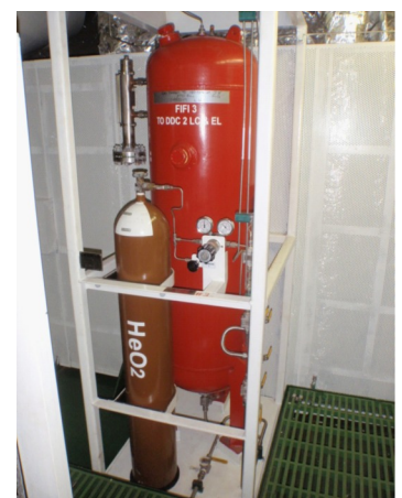
Volume tank & its pressurization sys.
