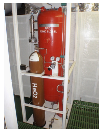
Volume tank & its pressurization sys.
