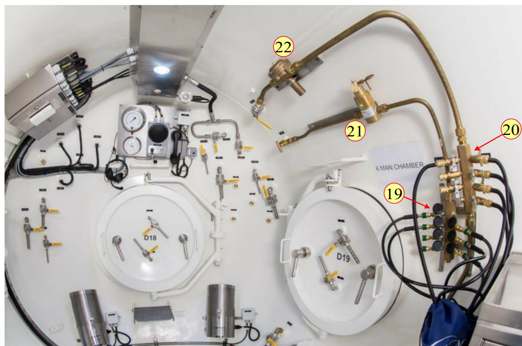
BIBS Inlet and outlet manifolds and valves. Also, note the valves an systems described previously
