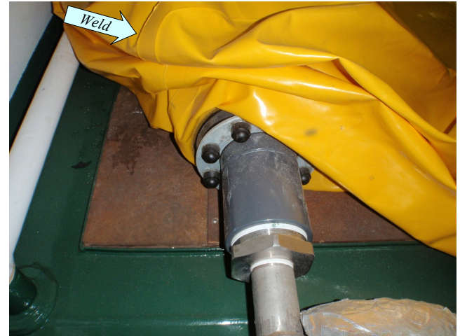
Exhaust connection. Also, note the welds of the tarpaulin
