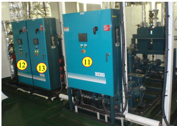
Electrical cabinets with Human Machine Interfaces
