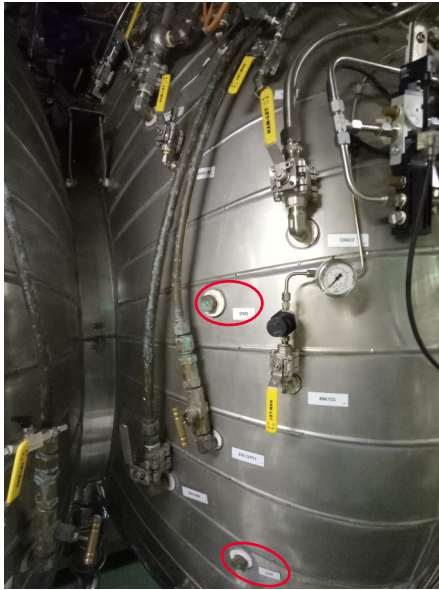
Marked hollow penetrators and their valves
