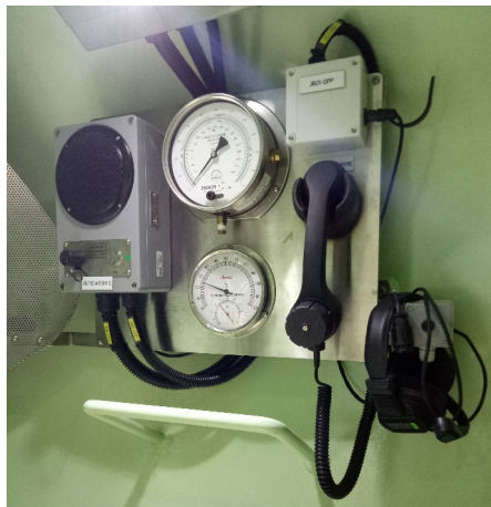
Communications grouped with gauges
