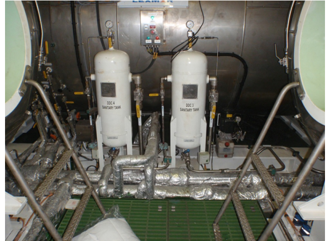
Sanitary discharge tanks (without specific protection)
