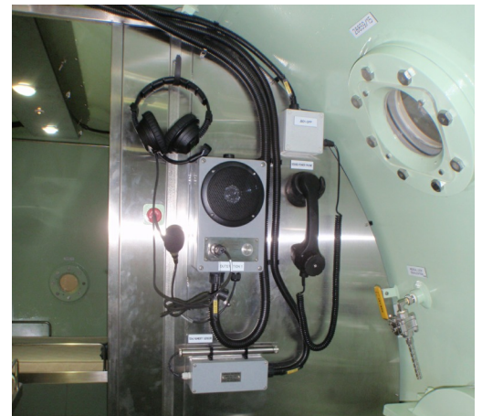
Communications not grouped with gauges
