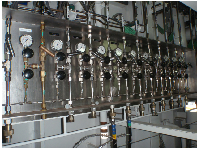
Gas charging panel - Note the oxygen line in yellow metal
