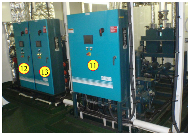
Electrical cabinets with Human Machine Interfaces
