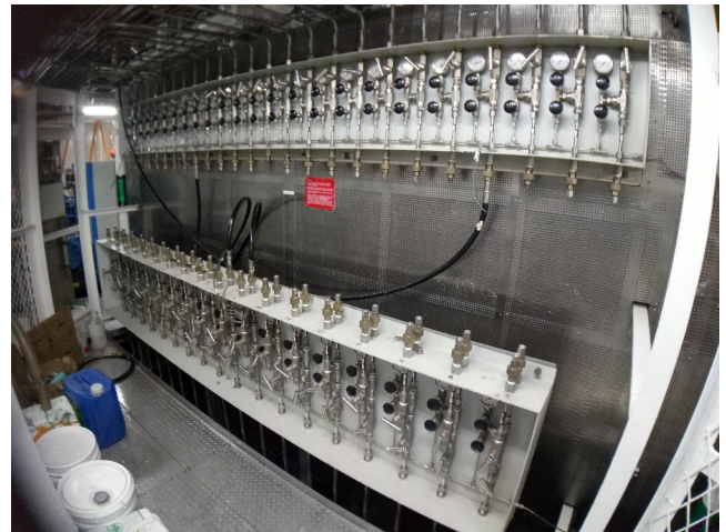
Gas storage panel (top) and gas distribution panel (bottom)
