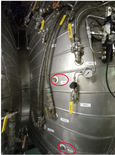
Marked hollow penetrators and their valves
