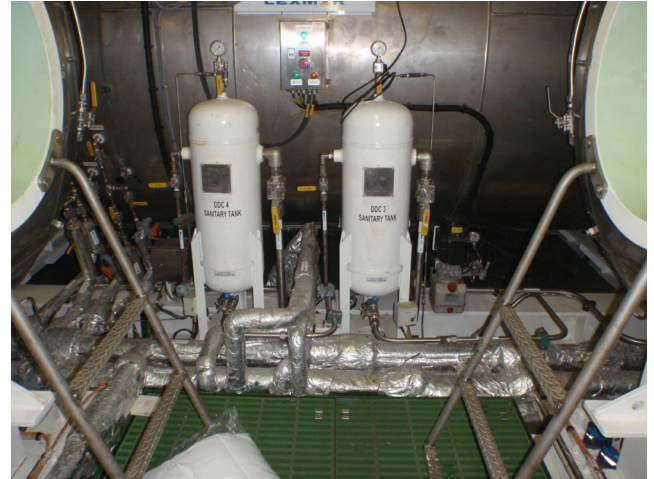
Sanitary discharge tanks (without specific protection)
