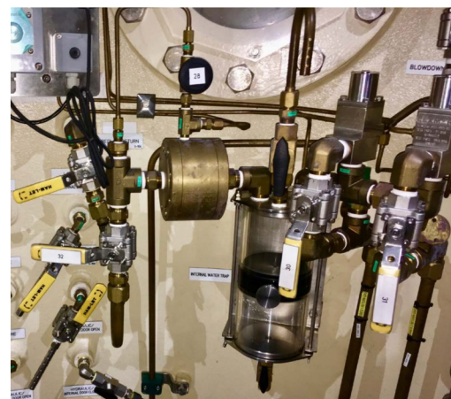
Back pressure regulator & water trap LEXMAR
