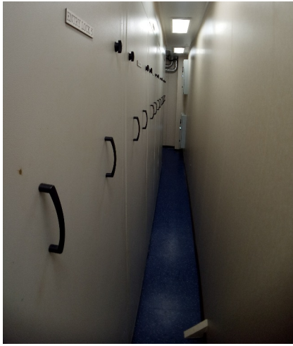
Corridor for access to the back of cabinets
