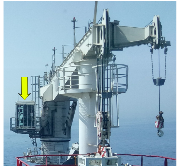
Control station in a cabin
