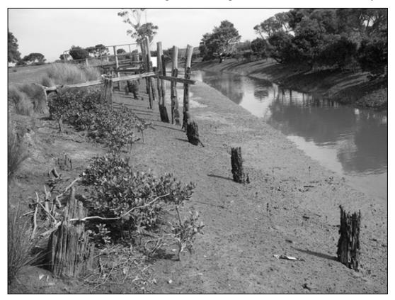
**Figure 42.** Remains of Dock Nine; note the advanced level of deterioration which suggests an earlier construction date than the others (Agnes Milowka 2006)
