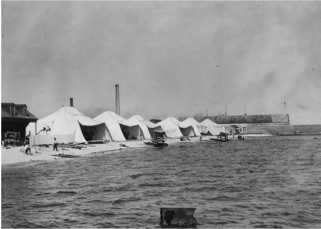
Figure 4. Canvas Seaplane Hangars at NAS Pensacola about 1914-1915 (1993.320.006; Courtesy the Emil Buehler Library)
