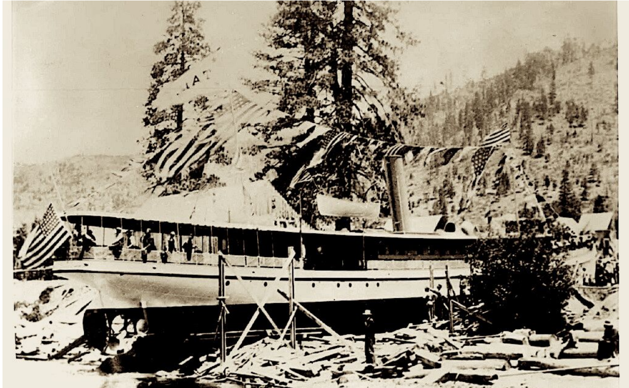
Figure 3. Preparing to launch the Steamer Tahoe. She was built at the Union Iron Works, disassembled, shipped to Glenbrook, Nevada, reassembled and launched on June 24, 1896. National Park Service photo.
