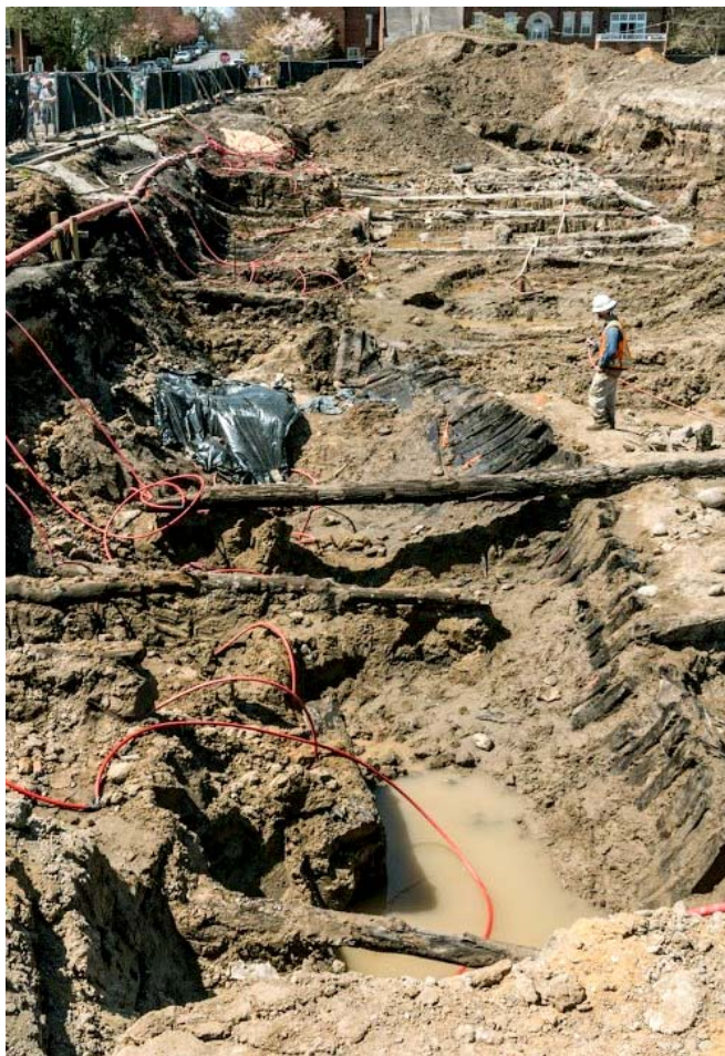
RTS Ship #3, unexcavated overview. Wharf cribbing in background and cribbing timbers cross the hull in middle ground. Courtesy of Alexandria Archaeology.
