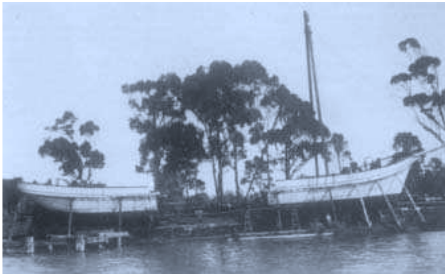
Figure 8.3 Lengthening of an unidentified vessel, at Harry Wood's shipyard, Launceston, Tasmania (reproduced by Orme 1988: 30, held by the Queen Victoria Museum and Art Gallery, Launceston)
