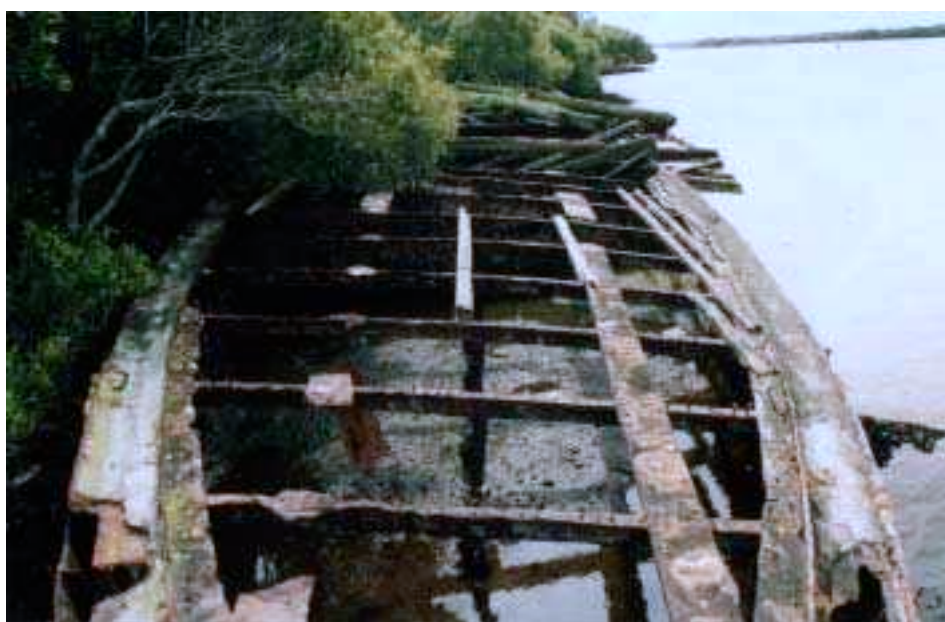
Figure 9.3 Remains of Federal at the Witts' Island Ships' Graveyard (New South Wales showing absence of paddle, boilers etc.. (Photo: Nathan Richards, 27/09/2001)
