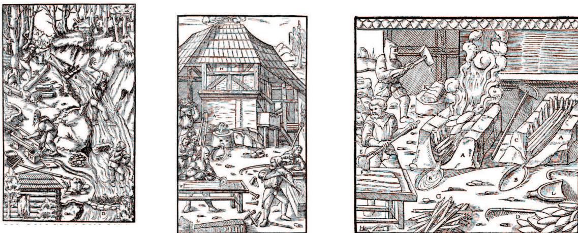
Figure 25 Plates from Agricola's De Re Metallica of 1556. From left to right, a: seifen extraction and washing in a diverted stream, book VII; b: pouring fluid tin on a thick copper plate in a lattice pattern; c: the lattice sheets are rolled with a wooden mallet, book IX (from: Hoover&Hoover 1950, 337, 415, 418).
