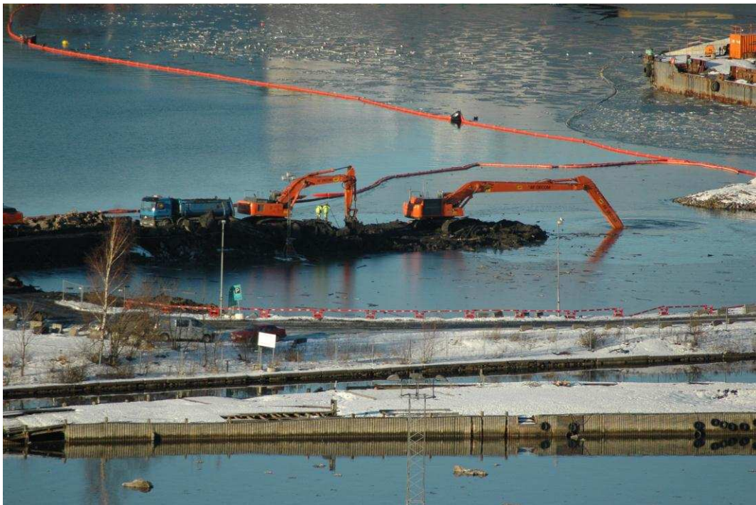
Figure 6: Dredging from the piers. Photo: Norwegian Maritime Museum.
