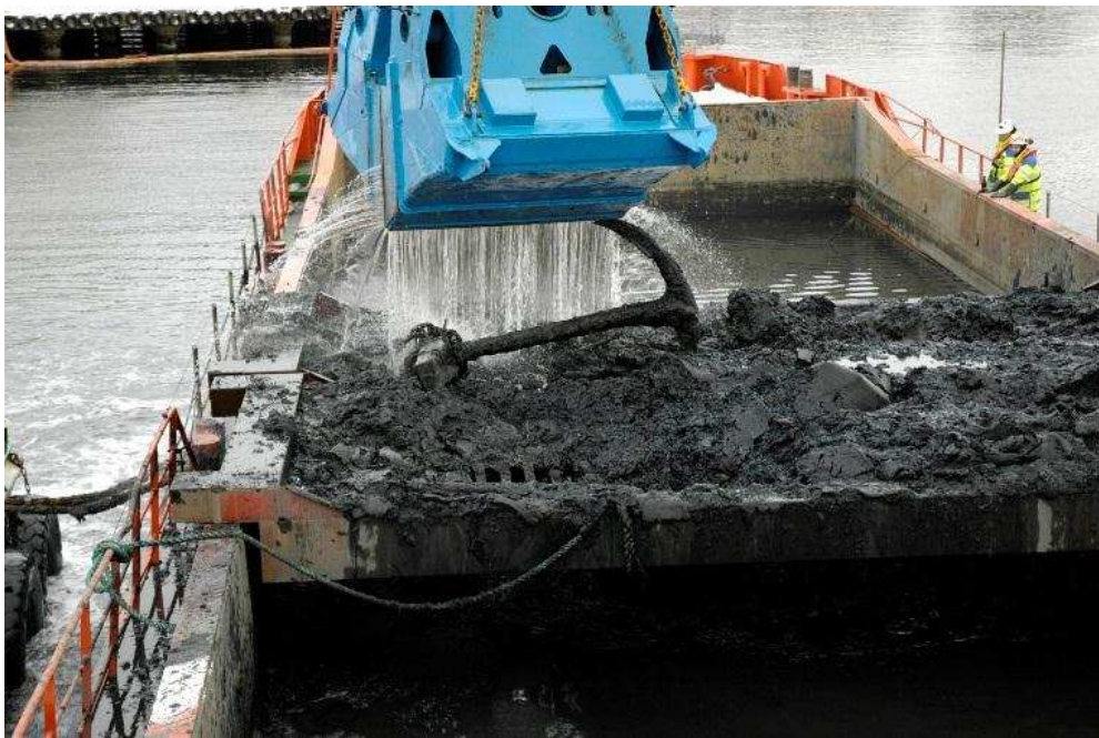
Figure 4: Dredging from barges in open water. On the custom made sieve a 19 th century anchor has appeared. Photo: Norwegian Maritime Museum.
