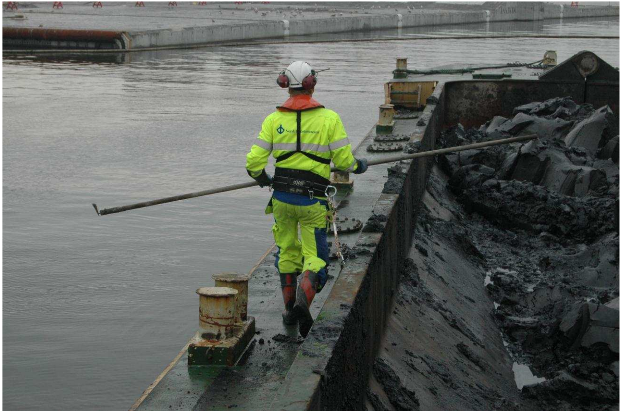
Figure 7: Dredging from barges in open water. Archaeologist on board. Photo: Norwegian Maritime Museum.
