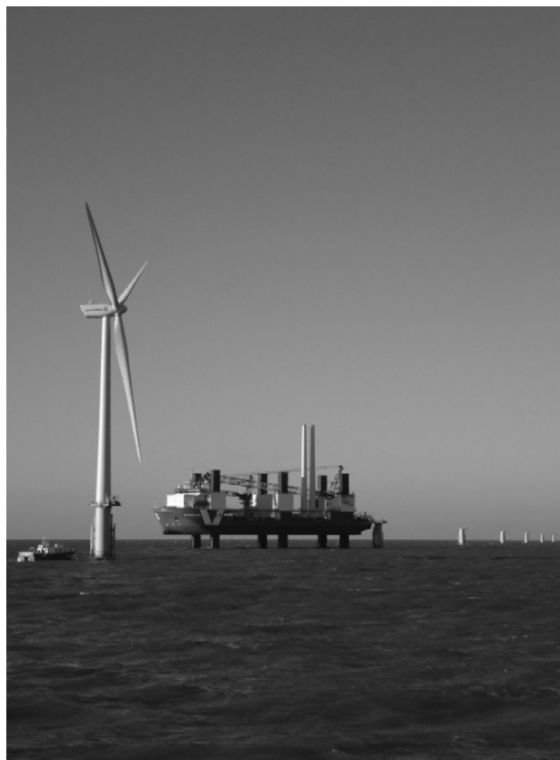
Figure 3. Wind farm under construction (Wessex Archaeology).
