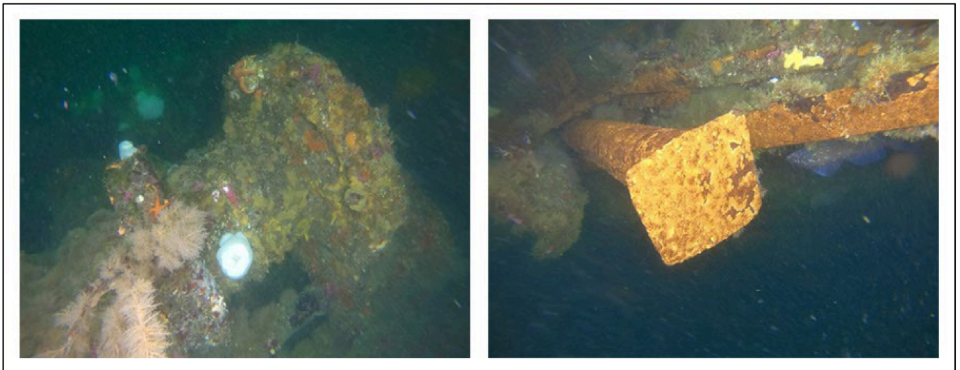
Figure 10. ROV imagery of SS Dellwood . (Left): Winch from the mast bed displaying significant calcareous concretion; (Right): Corroded deck beams.
