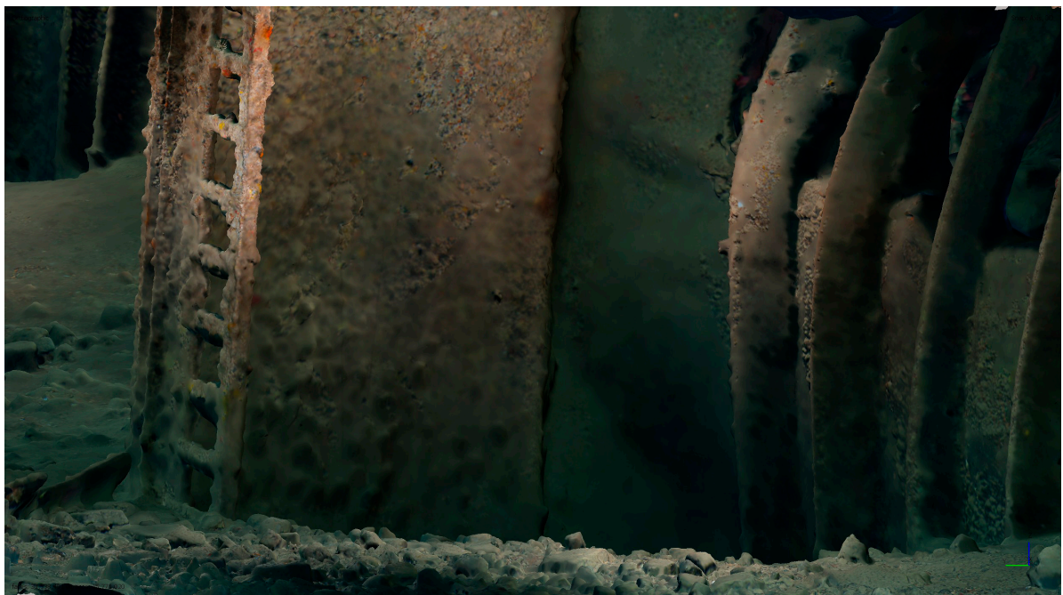
Figure 25. With the vertical ladder as a reference, the deformation of the watertight bulkhead ribs becomes apparent.
