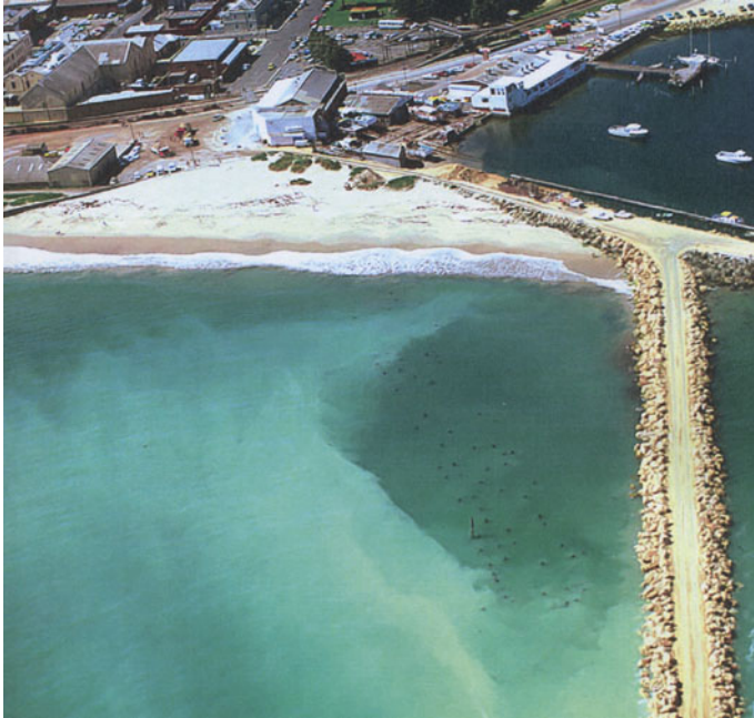
Fig. 3 The remains of the Ocean Jetty (the original part of the Long Jetty) with the development occurring alongside. The museum's team had left the water at this stage (WA Museum)
