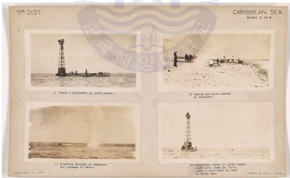
Fig. 35 Taking ashore and blasting the channel of Roncador Cay, June 1919 (NARA Identifier No 45704031).
