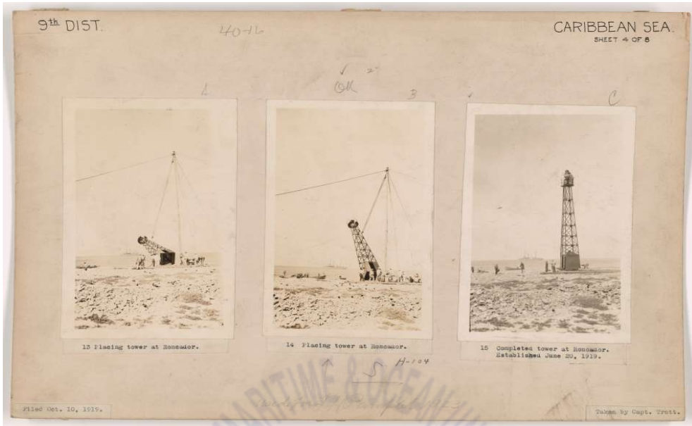
Fig. 34 Placing Tower at Roncador, June 20, 1919 (NARA Identifier No 45704039)
