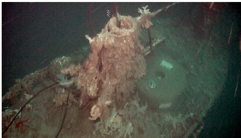
Figure 10. Clamp and cable arrangements for central anode pod connection to the conning tower. Note the replica hatch is in the “locked down” position.
