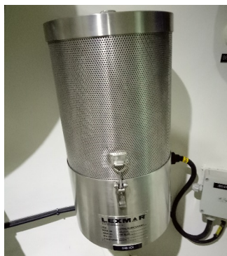
Scrubber installed vertically
