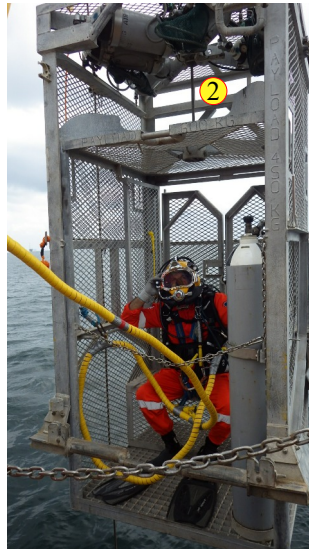
Deployment: The basket slides down in the standby diver's unit
