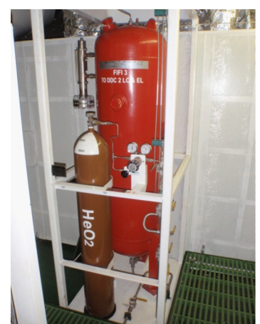
Volume tank & its pressurization sys.
