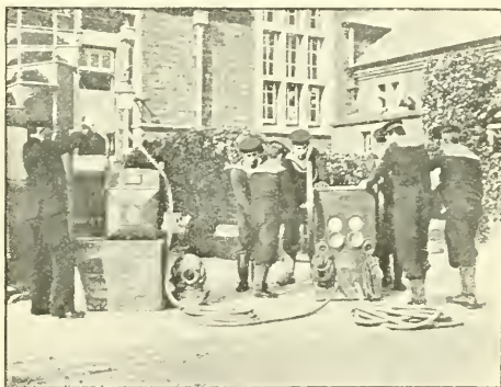
FIG. 33.—TESTING A PUMP BY METER AND SCREW CLAMP.
