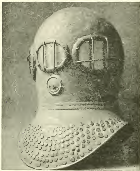
FIG. 12.—SIEBE'S FIRST DIVING HELMET.
