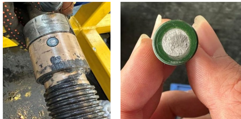
Figure 27. Shear pin damaged at a speed of 10 r/min.
