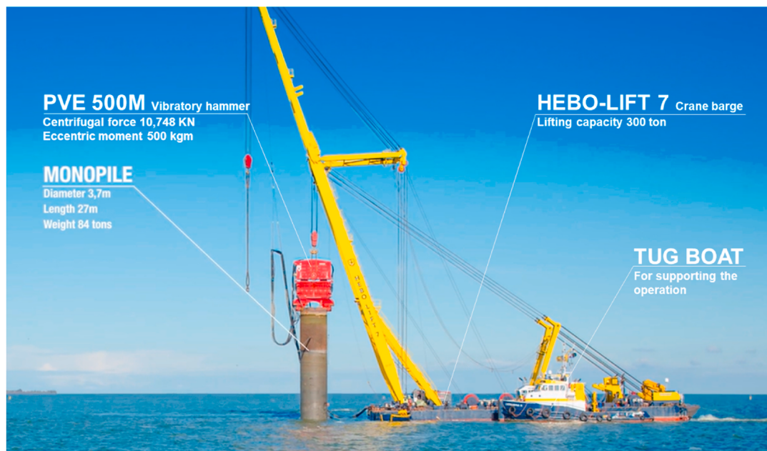
Fig. 1. System of monopile & vibro-hammer in decommissioning of Lely wind park (Dieseko Group, 2017).
