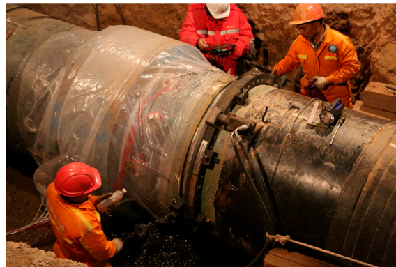
Figure 1. Installation of the insulating joint.
