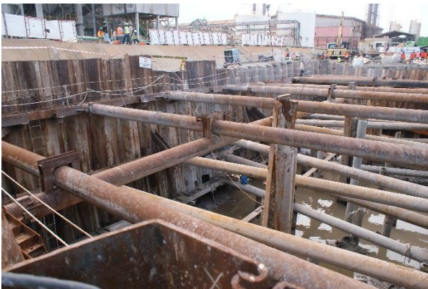
Figure 2. Excavation of Case 1 Project
