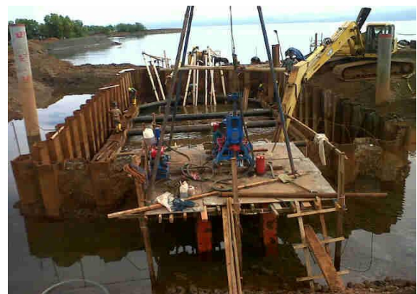
Figure 14. Excavation of Case 2 Project
