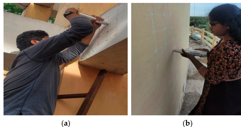
Figure 5. Rebound hammer test on the RCC water tank in Thirunallar: (a) beam element; (b) wall of water tank.
