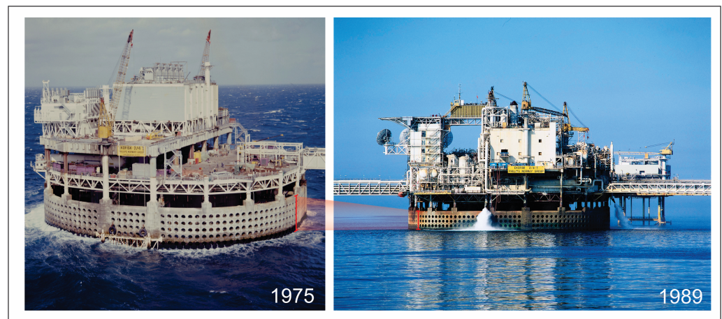
Figure 1. Subsidence recorded at the Ekofisk Platform over a period of 14 years: on the left, a photo taken in 1975 shows the platform shortly after its installation; on the right, the same platform in 1989 reveals significant changes due to subsidence (red marker). The picture is reproduced with permission. (Photo credits: Image 1975, ConocoPhillips/Norwegian Petroleum Museum; Image 1989, Husmo Foto/ConocoPhillips/Norwegian Petroleum Museum.
